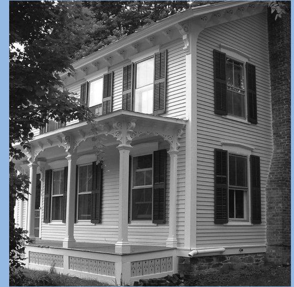
Home following completion of lead paint hazard reduction work.
